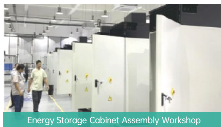
Energy Storage Cabinet Assembly Workshop
